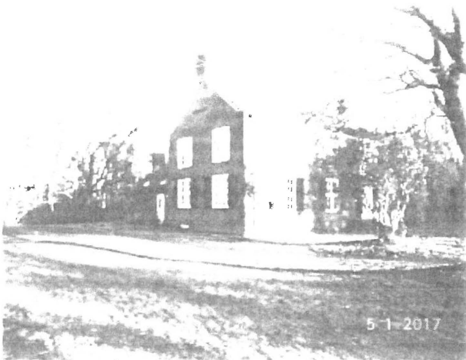
West side view
