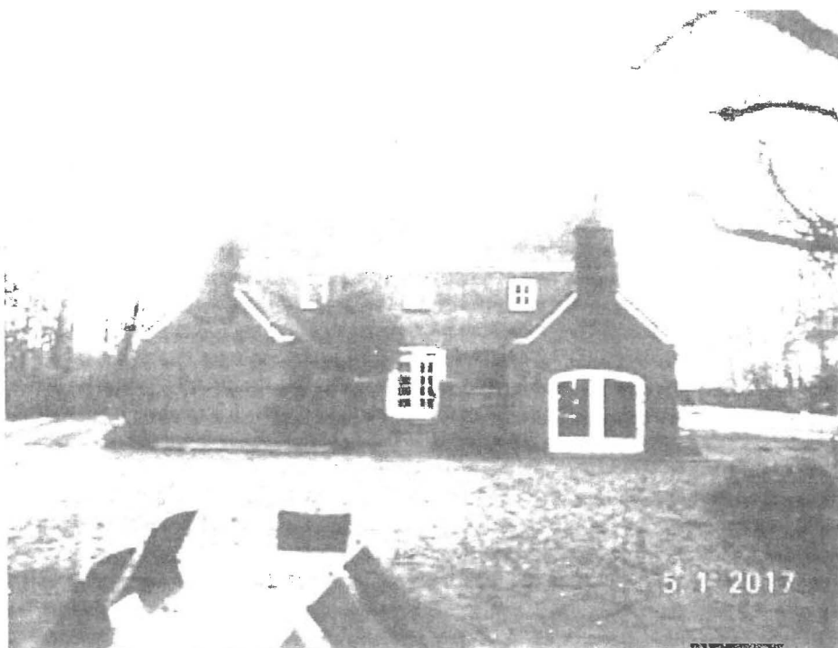
West side view
